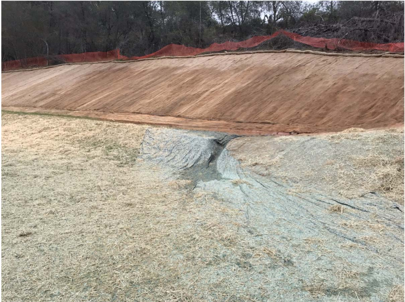
Pictured: New Erosion and Sediment Controls
